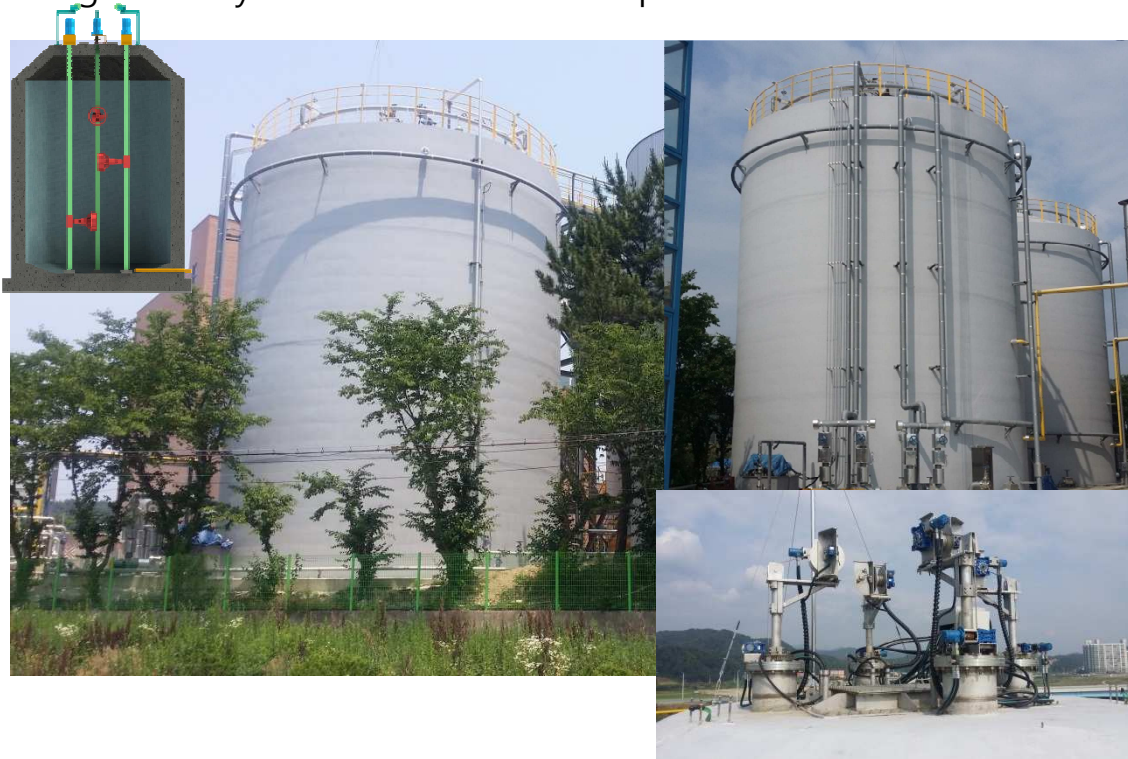
Ul-jin county environment recirculating livestock manure processing installation project construction
